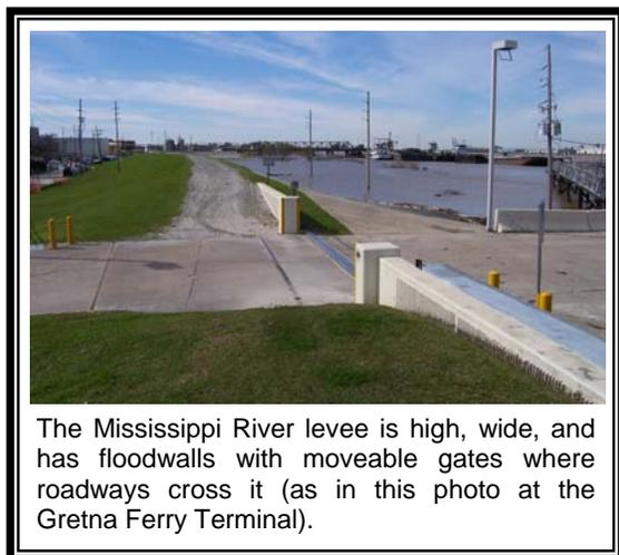
The Mississippi River levee is high, wide, and has floodwalls with moveable gates where roadways cross it (as in this photo at the Gretna Ferry Terminal).
