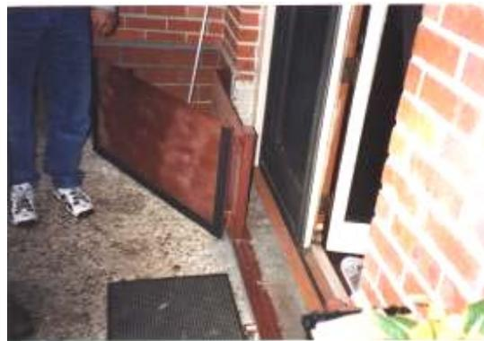
The same Baton Rouge home has a steel door with gaskets that seal when closed
