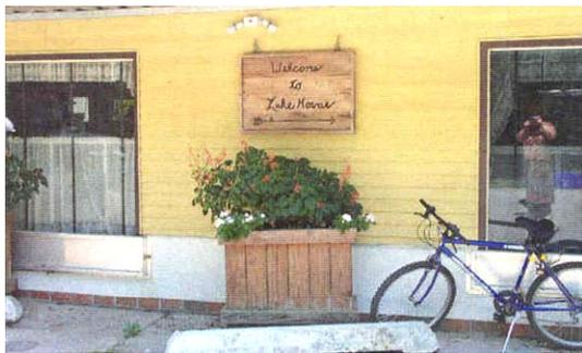
This dry floodproofed commercial building in Mandeville had the walls waterproofed and removable shields placed in the windows. While the measure worked for shallow flooding, the building was damaged by storm surge during Hurricane Katrina.
