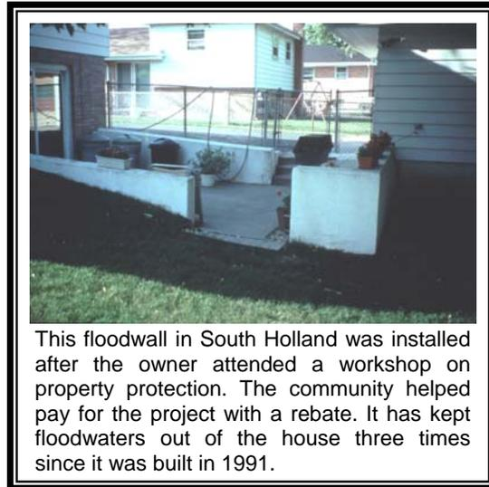
This floodwall in South Holland was installed after the owner attended a workshop on property protection. The community helped pay for the project with a rebate. It has kept floodwaters out of the house three times since it was built in 1991.
