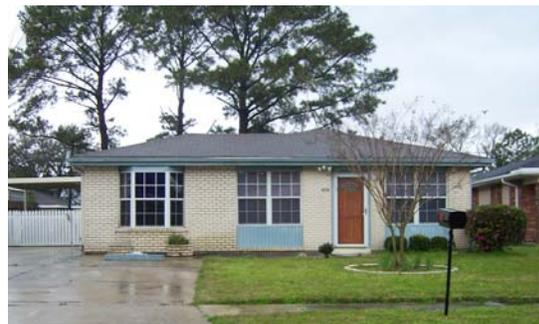
This Westbank home has permanent shields sealing the lower parts of the windows.
