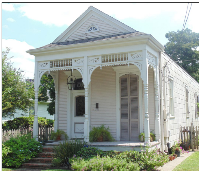
This Eastlake porch retains many of its original features, including brick steps, tongue-and-groove porch floor, turned posts, and decorative spindle frieze.
