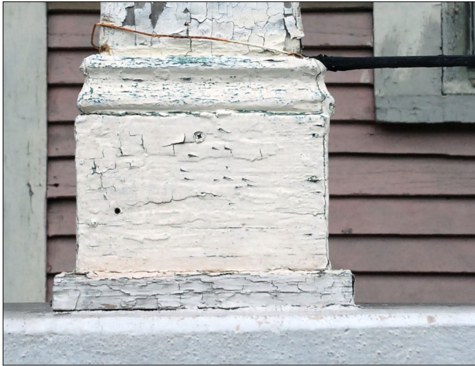
Example of maintenance: This porch column needs to be sanded, primed, and repainted.
