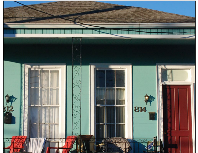
Several character-defining features have been removed. The porch beam has been covered with inappropriate vertical vinyl siding and the porch columns have been replaced with metal posts.
