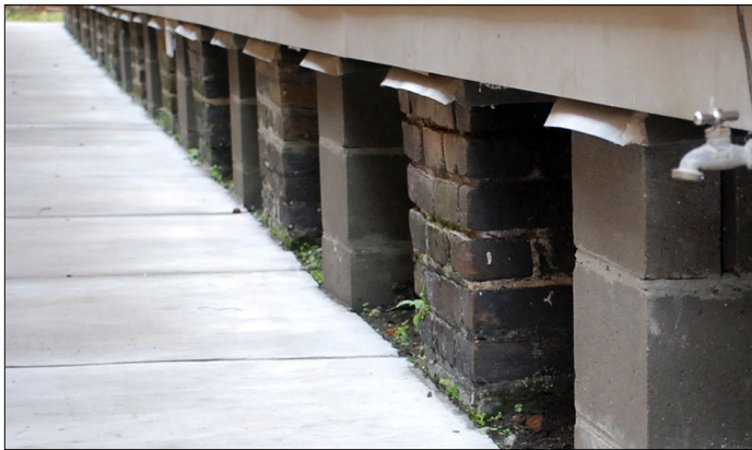
The foundation has been reinforced with new concrete piers placed between the original brick piers. Note that the piers have metal caps to prevent water and termite damage to the wood sills.
