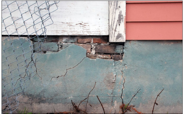
The stucco layer has been allowed to deteriorate, exposing the brick foundation beneath.
