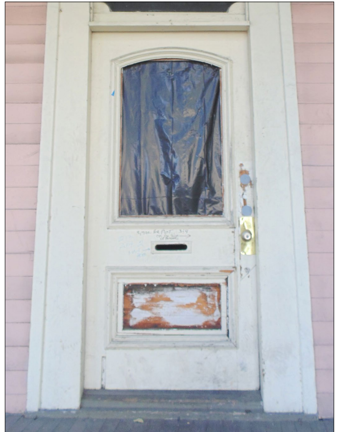
This historic door can be easily repaired with a fresh coat of paint and replacement of the segmental-arch light.
