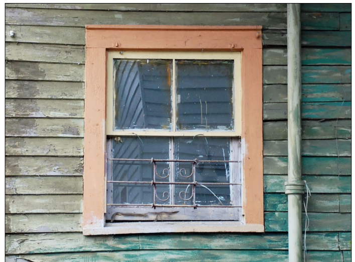
This double-hung wood window is in need of painting and sash/sill repairs.
