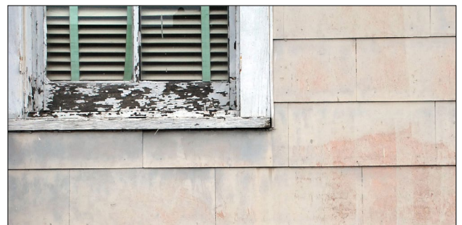
Asphalt shingles conceal the original wood siding beneath and should be removed if possible.
