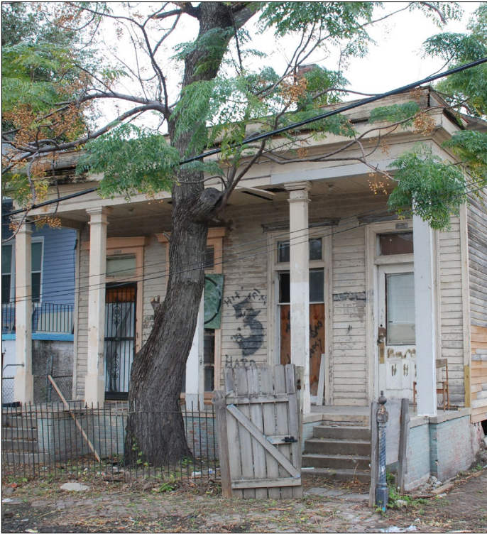
This porch retains a majority of its original elements. Although they are in poor condition, none are beyond repair.
