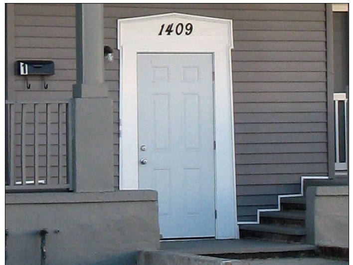
This modern door is inappropriate for its Greek Revival door frame.
