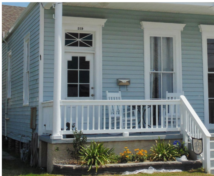
An example of a new wood porch and stair railing that is well proportioned, simply detailed, and compatible with the existing historic building.
