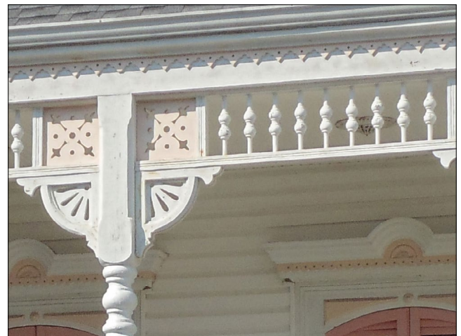
Piercework panels, a spindle frieze, spandrel brackets, and turned columns characterize the porch of this Queen Anne/Eastlake style shotgun.
