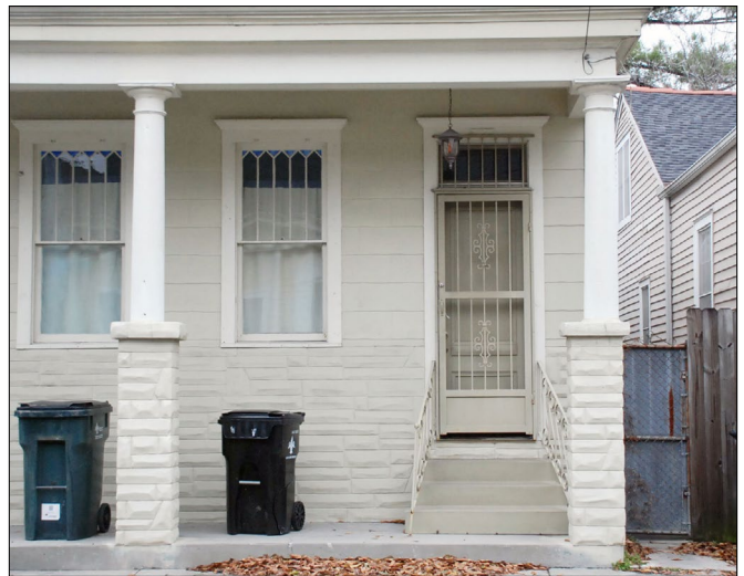
The original porch floor, balustrade, and steps have been inappropriately removed from this double shotgun.
