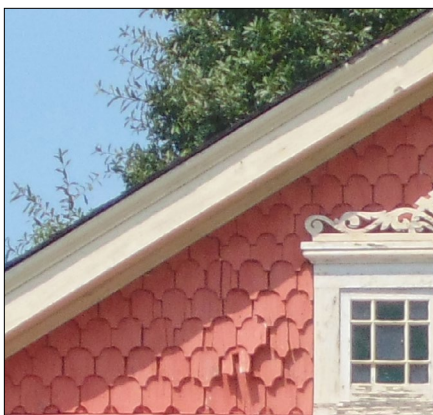
Sawtooth shingles in a front gable
