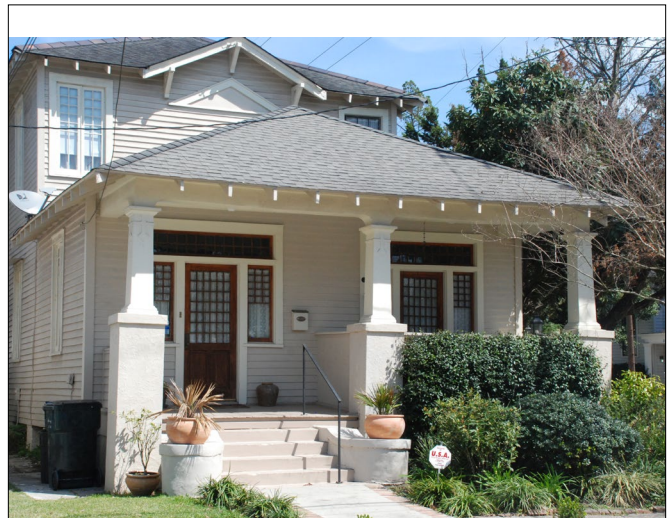
The steps to the entrance on the right were inappropriately removed when this residence was converted from a double to a single.
