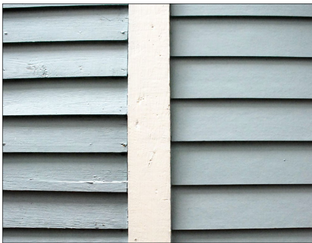
Smooth-faced HardiePlank siding (right) may be an acceptable alternative to wood weatherboards (left), especially on side and rear elevations.
