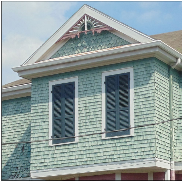
Wood shingles are defining elements of the Queen Anne style.
