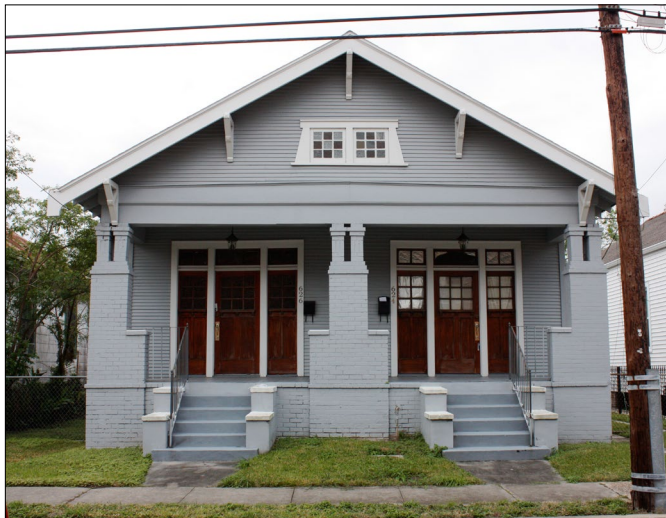
The two sets of steps are an important character-defining feature of historic double shotguns and cottages and should always be retained.
