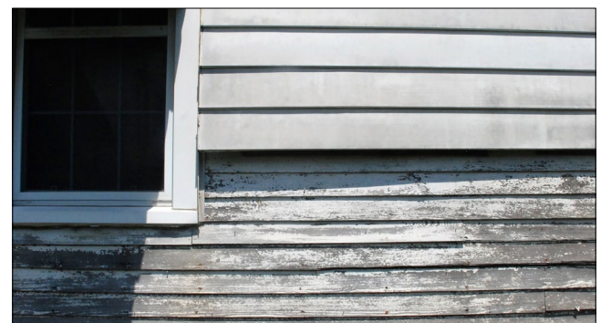
Aluminum siding was applied over the original wood weatherboards. It should be removed and the weatherboards restored.
