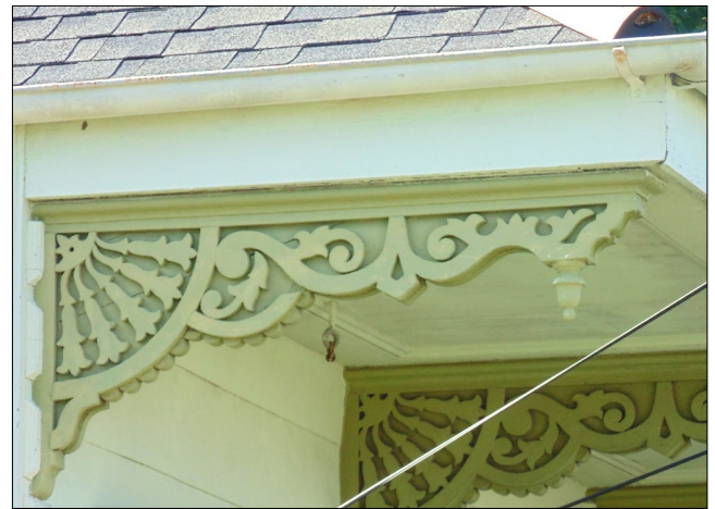
Milled brackets support the porch roof of a shotgun.
