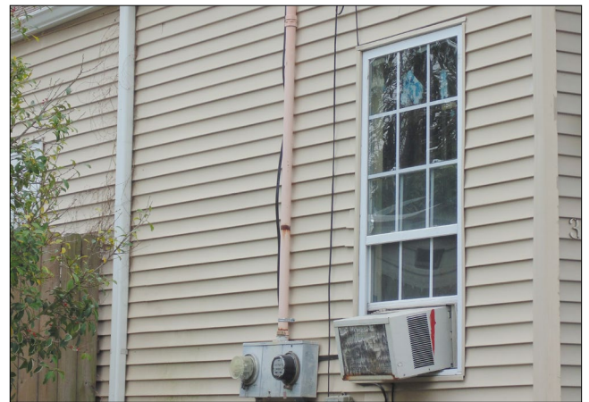
This vinyl siding swallows the wood trim around the window, concealing the casing's original profile.
