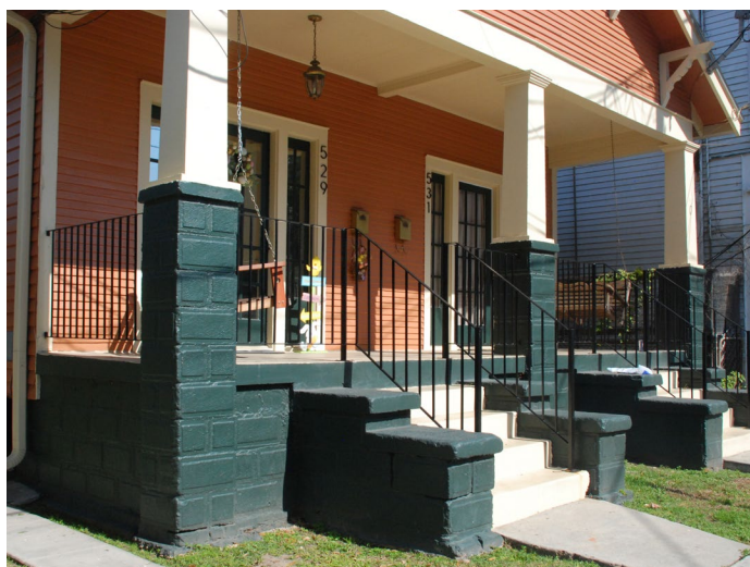
An example of a new simple metal porch and stair railing that is compatible with the existing historic building.
