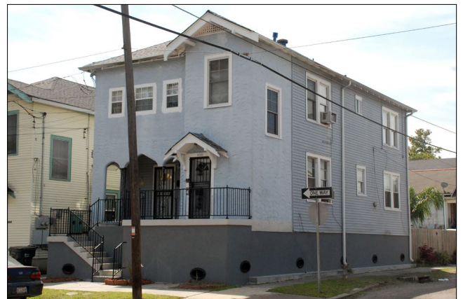
This two-story home was elevated approximately 6 feet above grade and the front porch was enclosed and finished with a layer of stucco. The foundation vents appear out of proportion compared to the prominence of the foundation.
