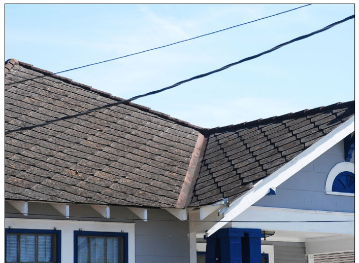
A well-maintained asbestos-shingle roof with copper flashing
