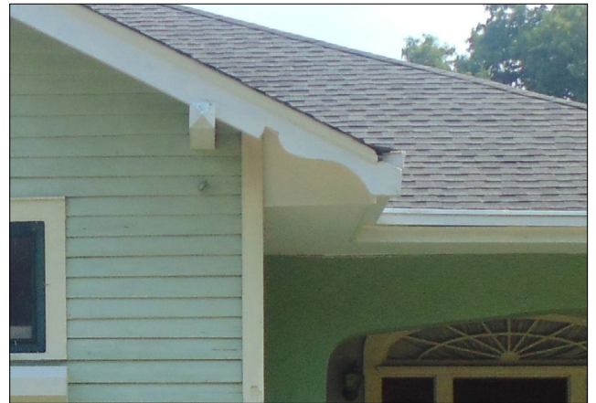
Enclosing soffits that were originally exposed jeopardizes a building's historic integrity.
