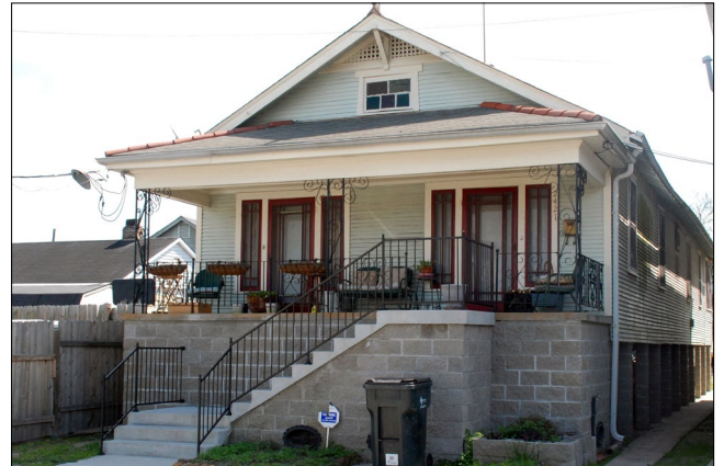
This Craftsman double shotgun was elevated more than 6 feet above grade, the concrete block chain wall was inappropriately left exposed, and the original front steps consolidated and repositioned.
