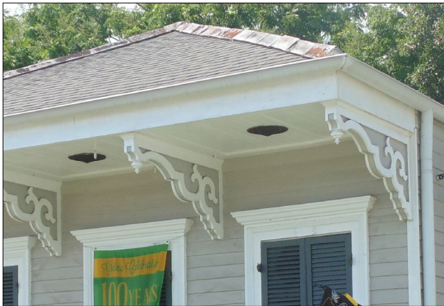
These half-round gutters and downspouts are appropriately placed and well maintained.
