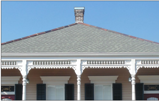
Asphalt shingles work well as replacement roofing material when blended with original elements such as terra-cotta ridge tiles.
