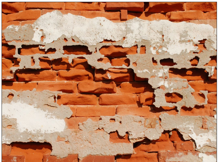
This is an extreme example of what happens when an inappropriately hard cement-based mortar is used on historic local soft brick. The brick wears away while the mortar, which should be “sacrificial” and fail first, remains intact.
