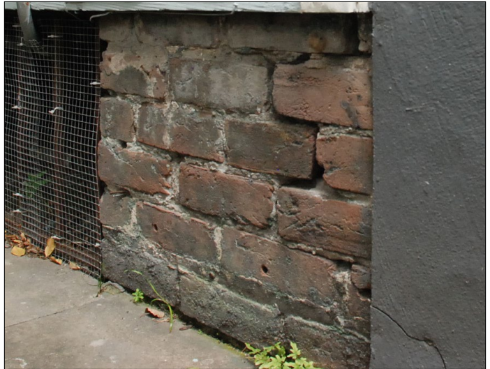
The mortar on this foundation wall is cracking and falling out in places. The brick is in need of repointing.
