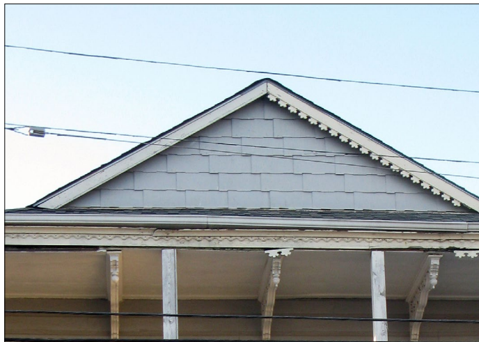
Example of replacement: The missing ornamental trim on the gable's left side should be replaced to match the trim on the right.
