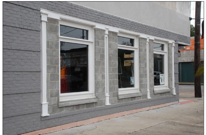
The original storefront windows of this two-story commercial building have been replaced with inappropriately sized window units and concrete-block fill.
