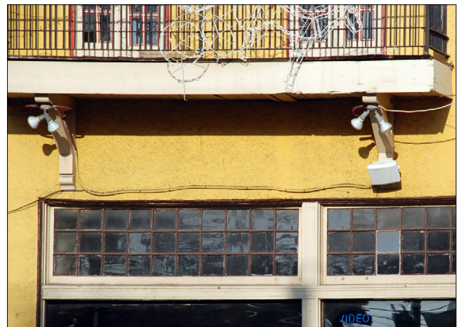
These flood lights with exposed wiring detract from the historic building's storefront.
