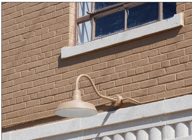
Gooseneck lighting is an appropriate way to illuminate a building's features.
