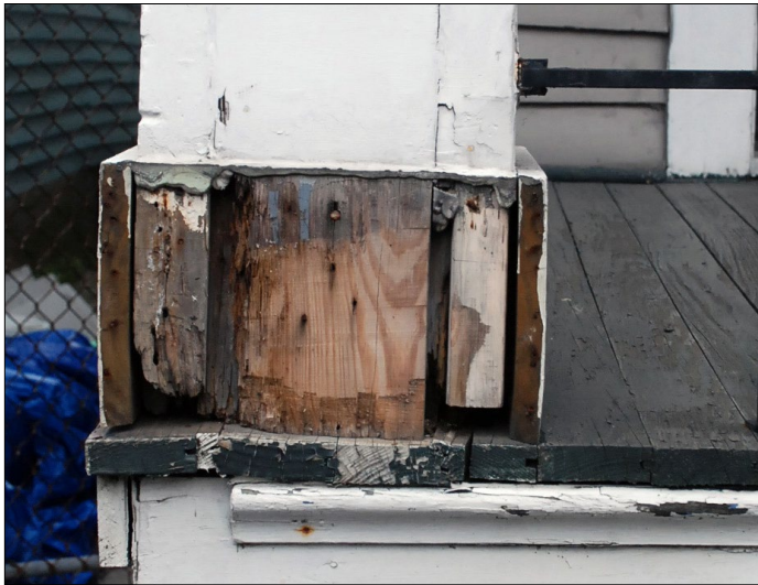
Example of repair: A piece of trim on this column base has fallen off and needs to be reattached.
