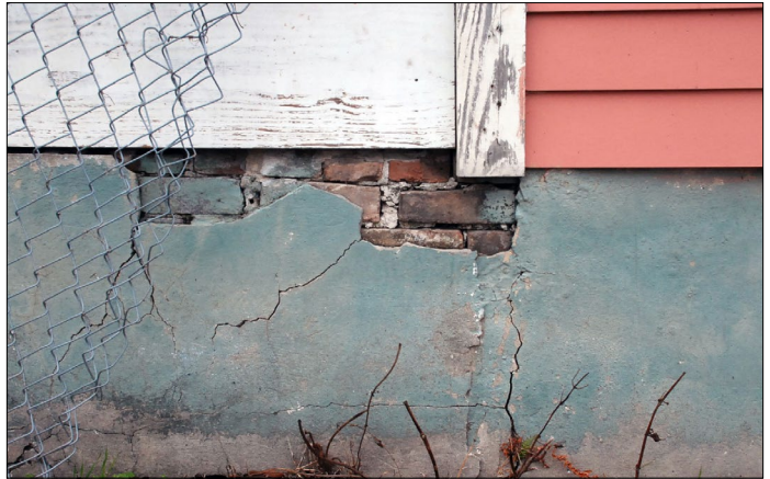
The stucco layer has been allowed to deteriorate, exposing the brick foundation beneath.
