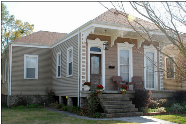
This bracketed shotgun has been minimally elevated. Landscaping effectively screens the foundation and provides a graceful transition to the ground plane.
