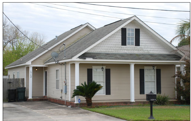
This new construction lacks the full-length windows, steps, and main entrance of a traditional front porch.
