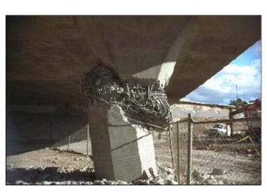
Figure A-15 Earthquake Damage Source: FEMA
