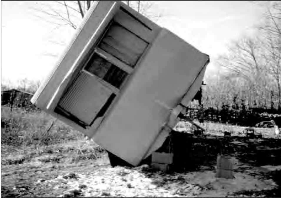
Figure 7-8. Failed foundation system that used masonry piers.
