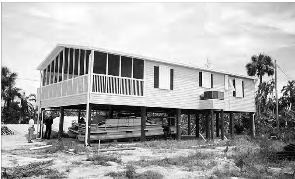
Figure 8-4. Manufactured home on a pile foundation.
