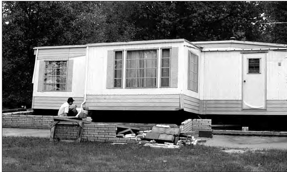
Figure 5-6. Failure due to sliding.
