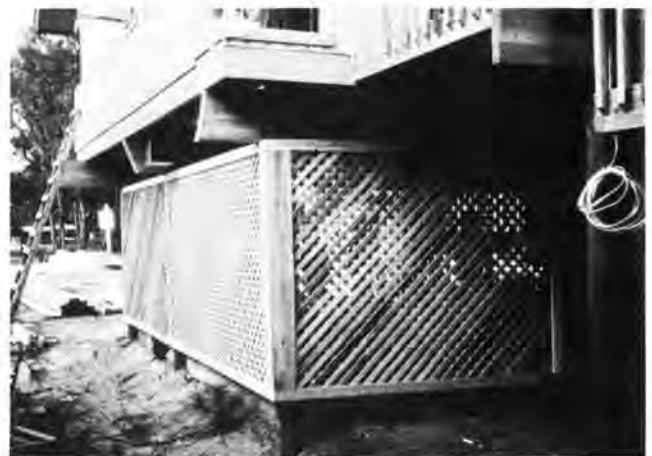
Figure 4.54. Breakaway Walls
