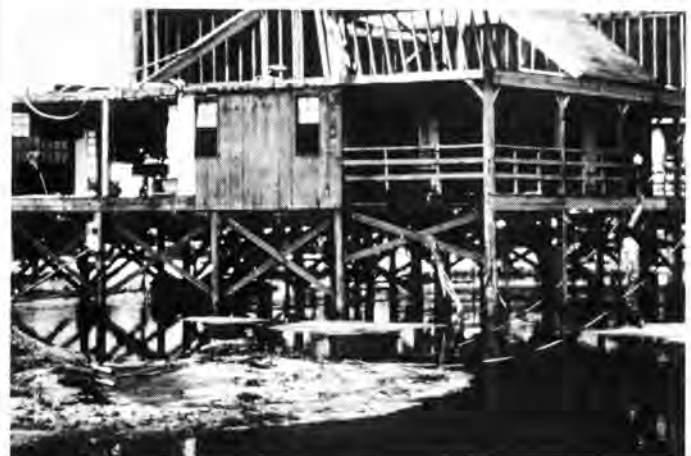
Figure 4.23. Diagonal Bracing
