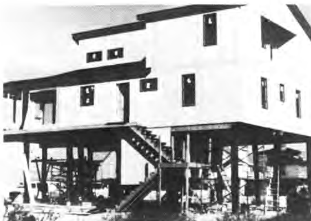
Figure 4.14. Pile Foundations
