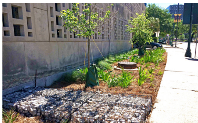
Bioswale at the New Orleans City Hall Parking Garage
