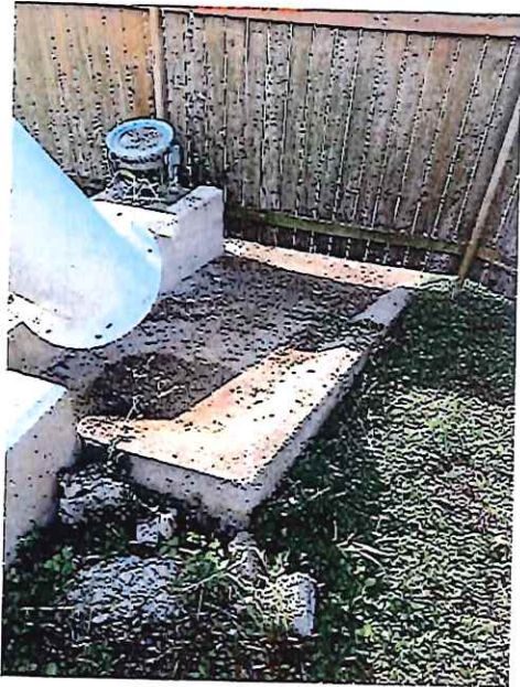
Splash Pad – good condition
