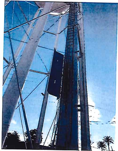
Exterior access ladder – good condition Ladder Gate/Vandal Guard – good condition
