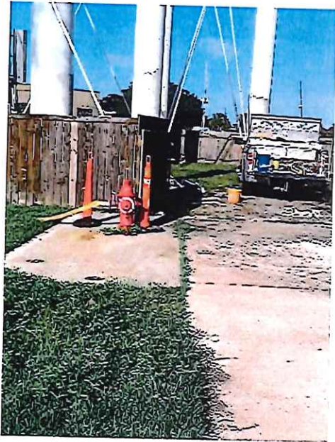
Water access via fire hydrant
