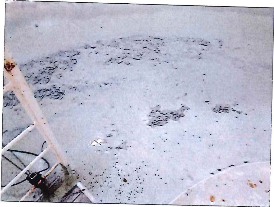
Interior Floor – Severe Pitting, paint failure and rusting
