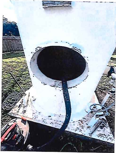
Riser manway – good condition Rusting around the opening
